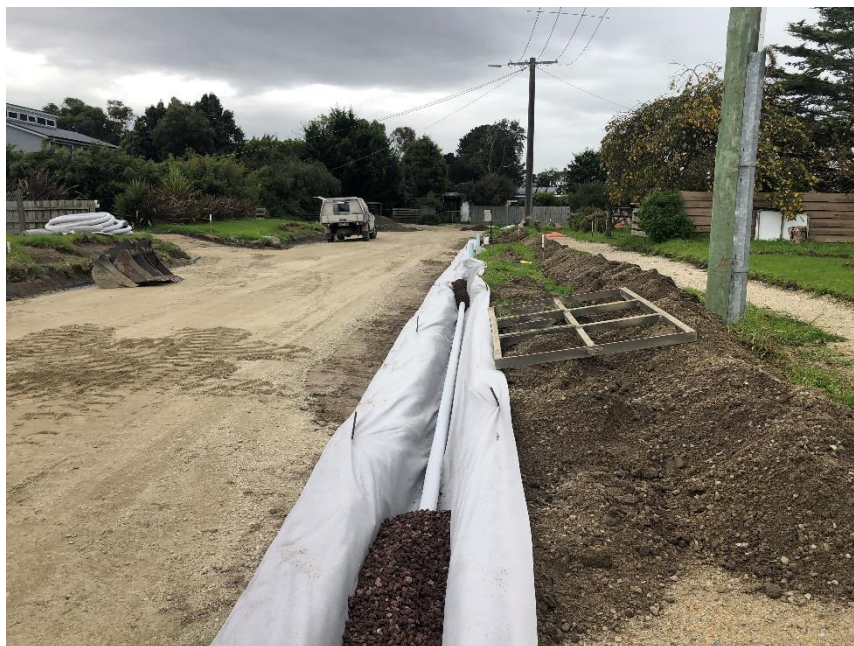
Aggy pipes being laid in Whiting Street
