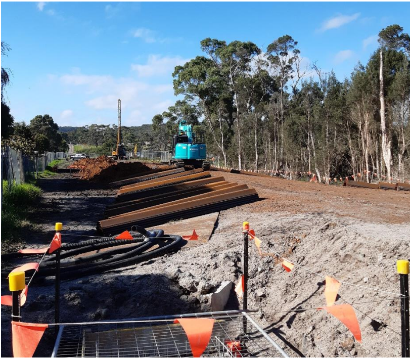
Construction of the swale and levee in the wetlands
