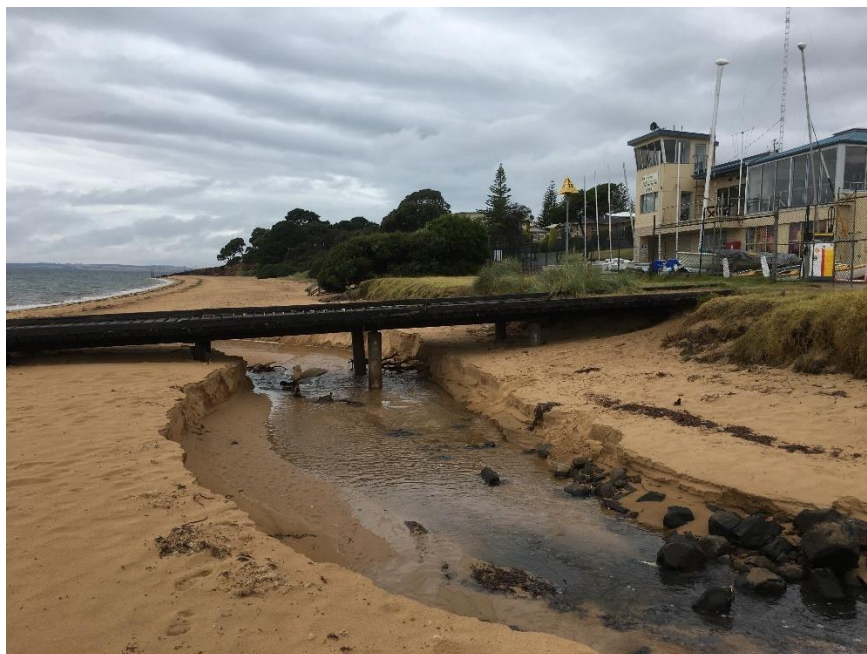
Figure 2-9 Beach scour by stormwater flow 29 Jan 2021.
