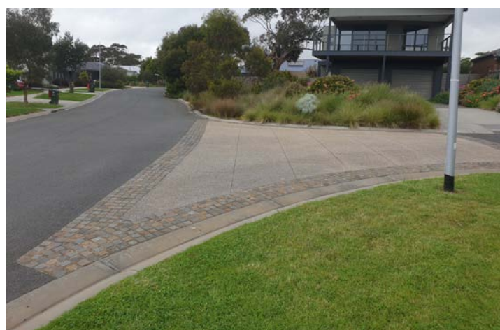
Intersection with threshold treatment, landscaping and swale drains in nature strip at Seagrove Estate Cowes.
